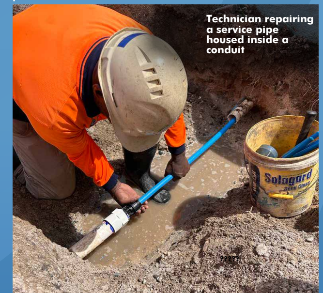
Technician installing a new service pipe at the corner of a driveway
